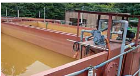
Cleanup of Contaminated Soil
